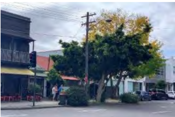
Figure 26. 88, 86, 84, 82, 80 and 44-78 Rosehill Street, Redfern
